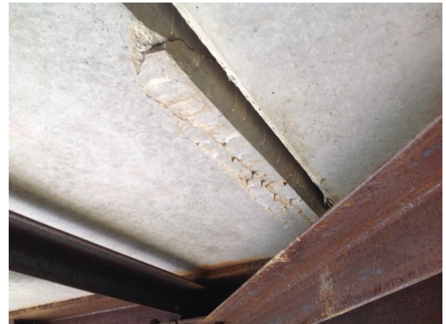
damage noted to first and second panel on right approach
