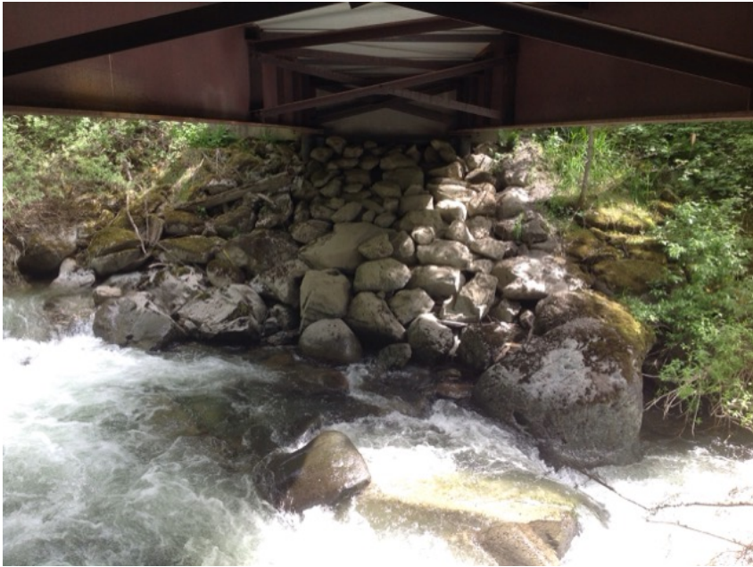
Left Bank Abutment when facing downstream
