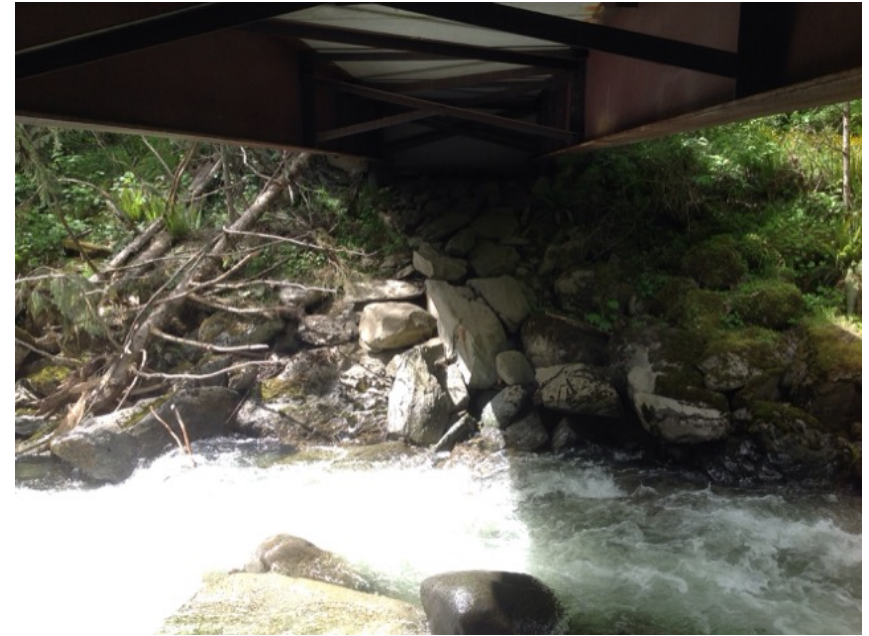
Right Bank Abutment when facing downstream
